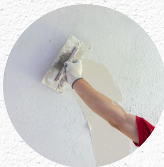
Internal plastering of walls
