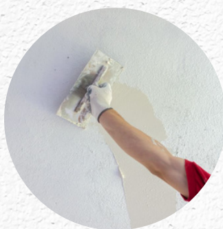
Internal plastering of walls
