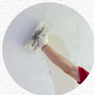
Internal plastering of walls
