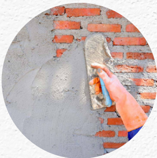
External plastering of walls
