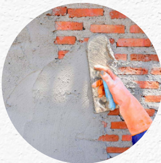
External plastering of walls
